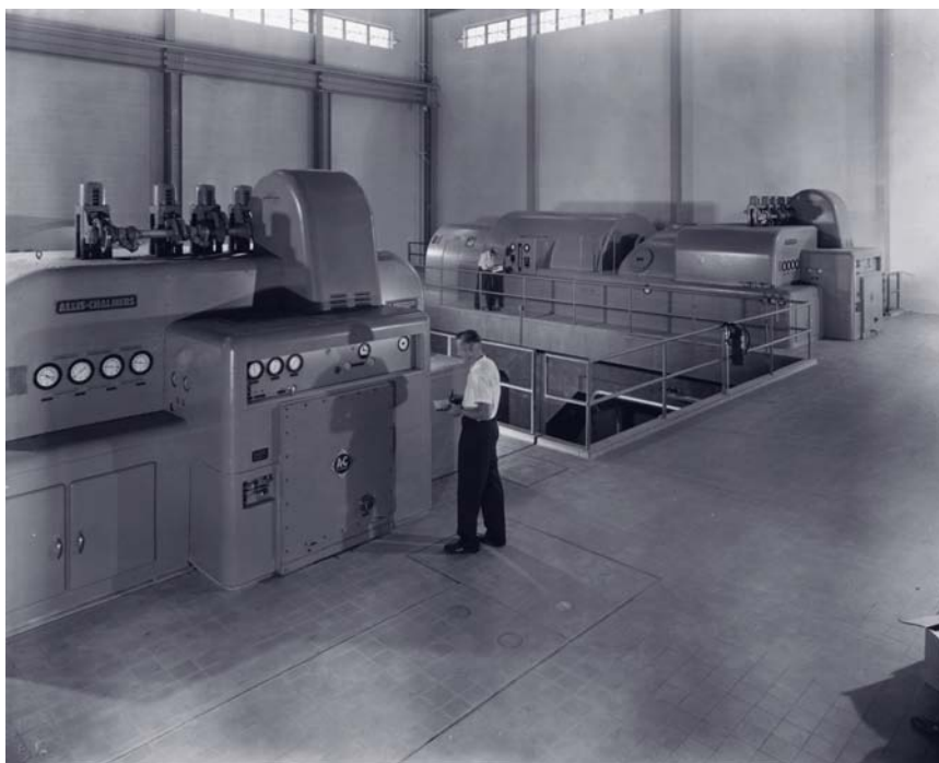
IP&L engineer Phil Hansen checks the output of one of the Allis-Chalmers turbine-generators at the Blue Valley Power Station, circa 1960.
